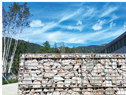
Building "gabion wall" with waste stonework
