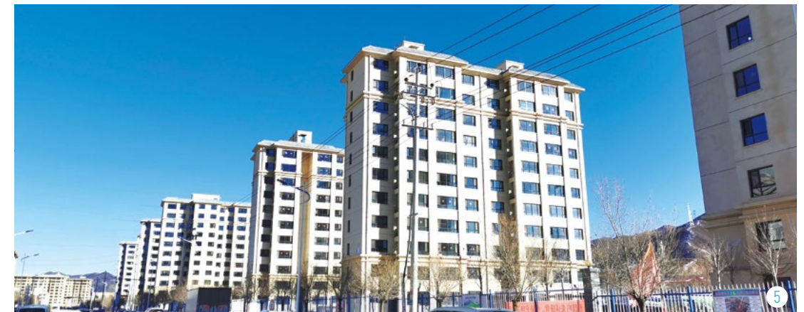
1. Resident representatives discuss the land requisition and relocation plan 2. Residents representatives participate in site selection and architectural design 3-5. Living environment after relocation
