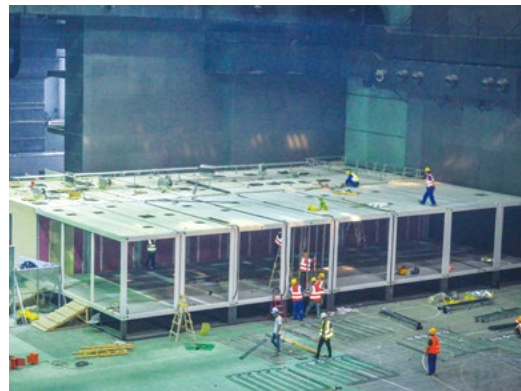
Athletes' dressing room in the construction of prefabricated container in National Indoor Stadium
