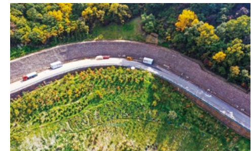
The stages of the topsoil stripping and reuse in the Yanqing Zone
