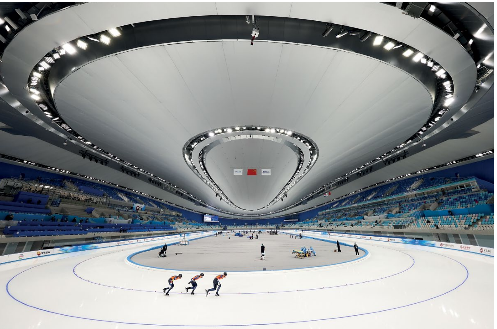
The National Speed Skating Oval is one of four Beijing 2022 venues to benefit from natural CO 2 refrigeration systems.
