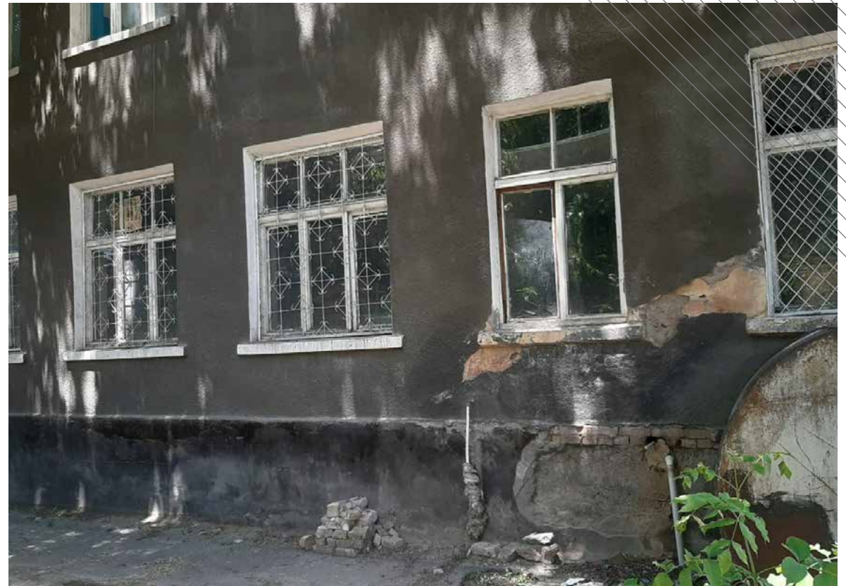
Special projects funding helped the NOC of Tajikistan to renovate the Ibrahim Hasanov Sports School
